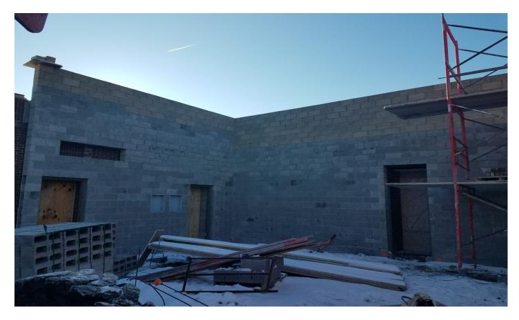
Construction of the new Main Office/ Secure Entrance has begun. This is the new fire wall separating the new space from the existing building. The new Exterior walls will be underway next week.
