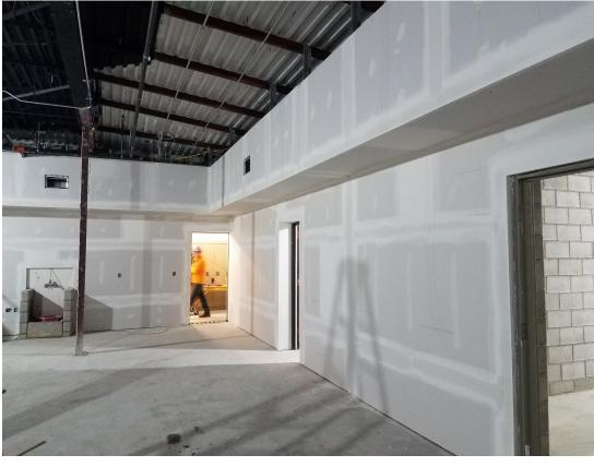
Drywall is being completed in the Band Room and ceiling grid and tile is being installed in corridors and rooms.
