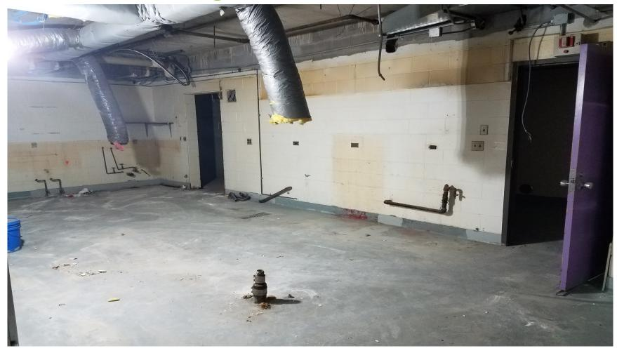
The existing kitchen equipment has been demolished to make way for the new serving/kitchen area. The next step is to remove the floor and select walls to start the underground work for the new serving/kitchen layout which will be much more student and staff friendly.
