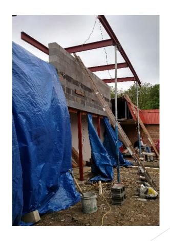
The steel for the new roof being installed.
