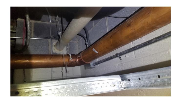
Installation of the 4" copper to replace the original galvanized pipe.
