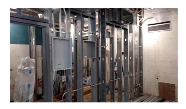
The new Administration offices new fire and time boxes along with all electrical roughed in. Plumbing trench which ties in the drain for the new bathroom re-poured.
