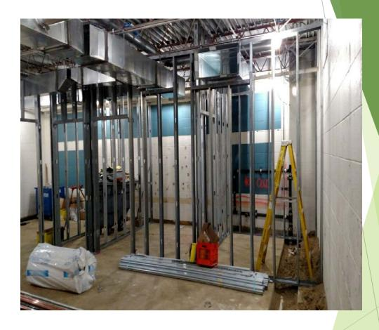
The new Administration office completely demolished. Electrical, mechanical, plumbing and carpentry roughin has been completed in the new Administration office.
