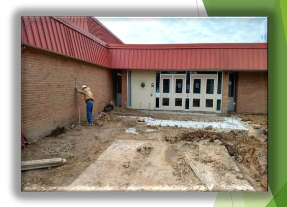
Pouring concrete for new footings and piers for new secure entrance.
