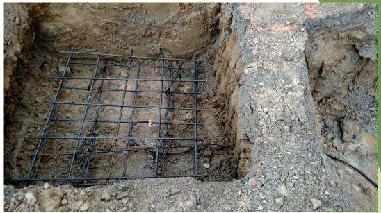
The new foundation for the new secure entrance with the bonding attached to it.
