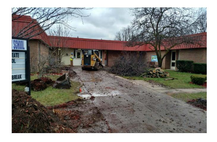
Starting the clearing of debris and concrete for the new secured front entrance at Wood Creek Elementary School.
