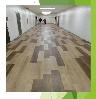
New fire-rated grout filled doors and fire-rated glass complete. Flooring in corridors and cafeteria. We will be wrapping up base on 2<sup>nd</sup> shift.
