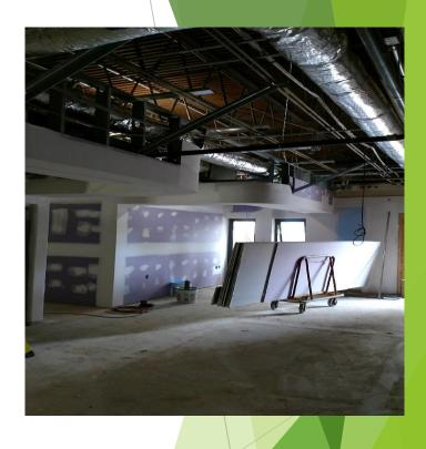
Main office door new frames toothed into existing masonry walls. New gyp walls and cmu wall constructed. Drywall radius soffits done. Drywall finishing underway.
