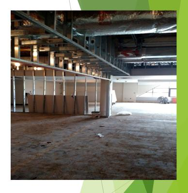
During these few weeks, work is still in progress in the Media Center. Metal stud framing and Electrical have been some key issues.
