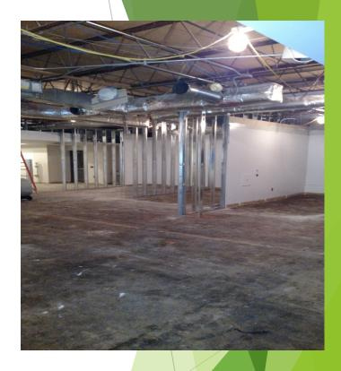
And with the "New" comes the installation of metal stud framing, air duct lines and electrical services being relocated.
