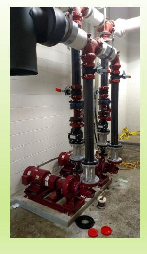
Upstairs in the Mezzanine, the new chiller pumps are getting brought up on line. The chiller is set and getting piped as well.
