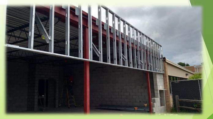
Exterior soffit/parapet framing construction.
