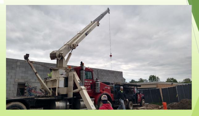
Steel is underway. Connelly Crane is erecting a column.
