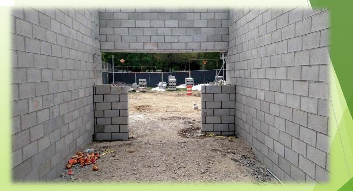
Navetta Masonry has begun to set the entrance Block walls. They will finish once steel is erected.
