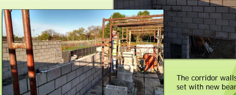
The corridor walls have been set with new bearing plates.
