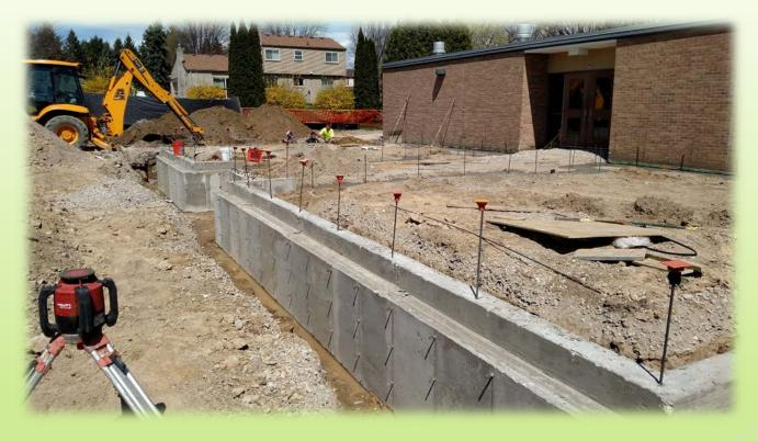
Finished pier walls with brick ledge and resteel.
