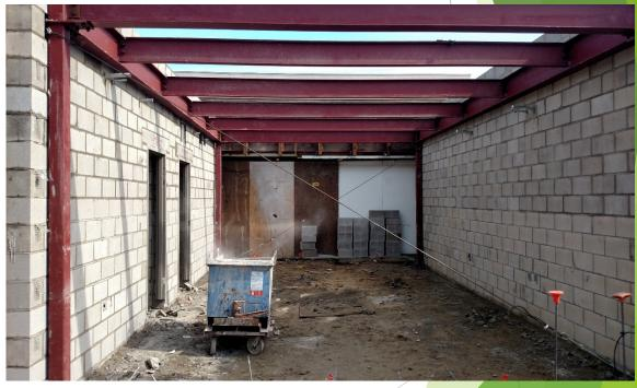
The new steel framing has been installed at the two additions and the masonry is ongoing.
