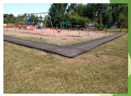
The base layer of asphalt is in place and the play area and the new walk path around the playground is installed.
