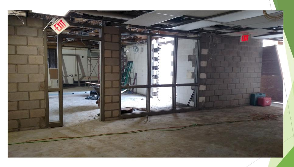
The new office area is taking shape as the new corridor wall and interior door openings are constructed.
