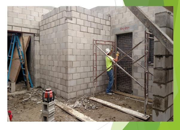
The new secure entrance at the main office is under way, the mason is laying block and setting bearing plates for the new steel.
