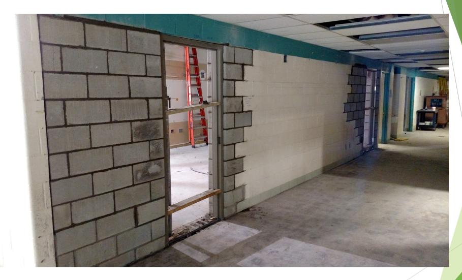
Newly installed hollow metal frames in masonry walls.
