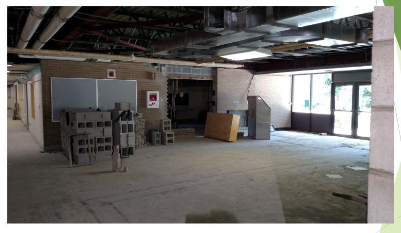
RTU #1 duct supply lines and the new entrance. CMU walls for secure entranceway are starting this week.
