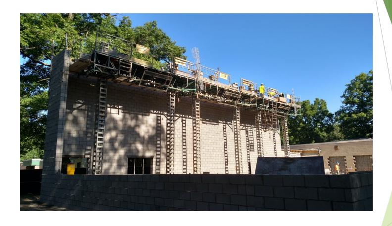
The Gym's west masonry wall is at full height. We continue with wall construction for the upcoming steel placement.
