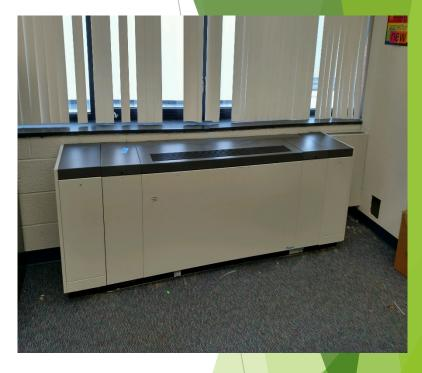
18 classrooms have been renovated with fresh paint new flooring and new furniture. 10 new unit ventilators were installed in the second floor classrooms over break; existing unit ventilators in other areas are being updated with new control valves.
