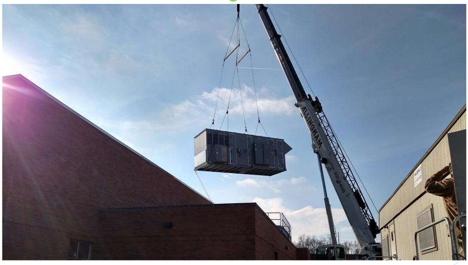
The new dehumidification unit for the pool has been set. Duct work on the roof to the pool area can now proceed.
