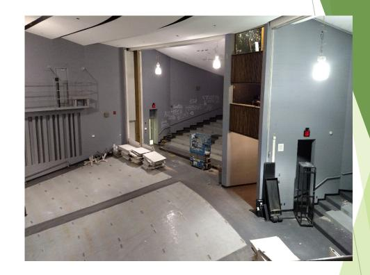
The auditorium project started on December 22; the seating has been removed, the folding partitions have been demolished, the fire curtain has been removed and electrical demolition is underway.
