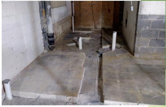
The gym locker room demolition is complete and the new underground plumbing has been installed.
