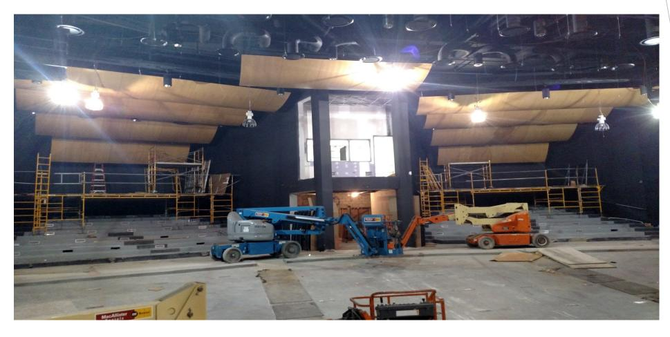
The painting in the seating area has been completed and the acoustical clouds are being installed.
