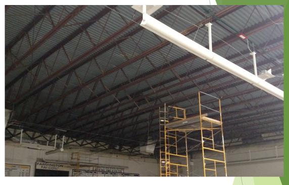
The pool has been drained, scaffolding has been erected, and the suspended ceiling has been removed.
