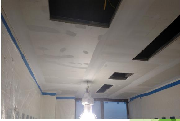
The drywall ceilings in both bathrooms need the finish coat then sanding. Fixtures and partitions should be in this week.
