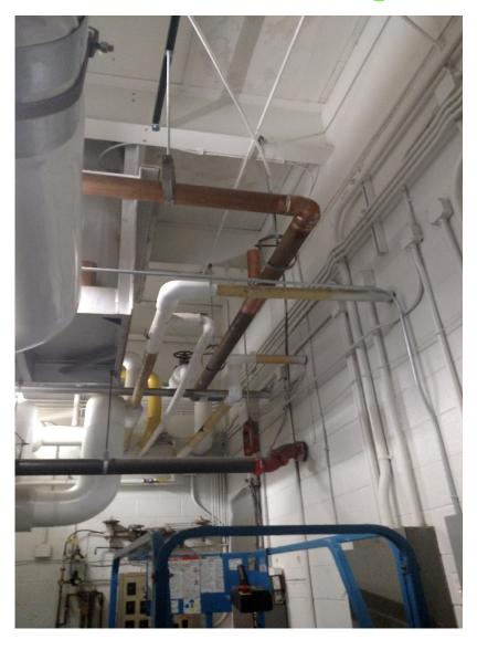
The replacement of the domestic water line has been in process here some of it can be seen in the boiler room.
