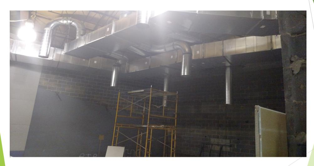
The new supply at the left rear wing has been completed, just the diffusers remain.
