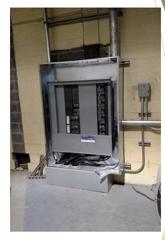
The new auditorium lighting controls are being installed as well the replacement of the auditorium power distribution panel.
