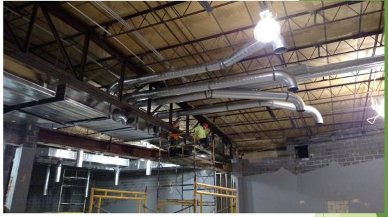
The new duct work is underway in the auditorium, here you can see where the diffusers will be located, these locations will be between the acoustical clouds when complete.
