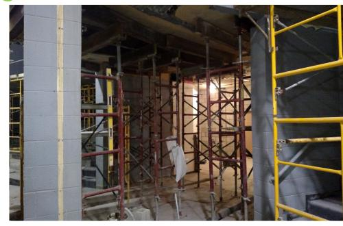
In the Auditorium the control tower has been shored to allow for the demolition of support walls to allow for the install of new steel.
