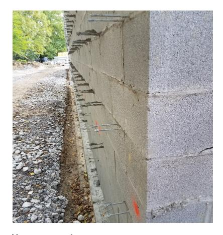
North wall of addition: Wall is ready to accept face brick.
