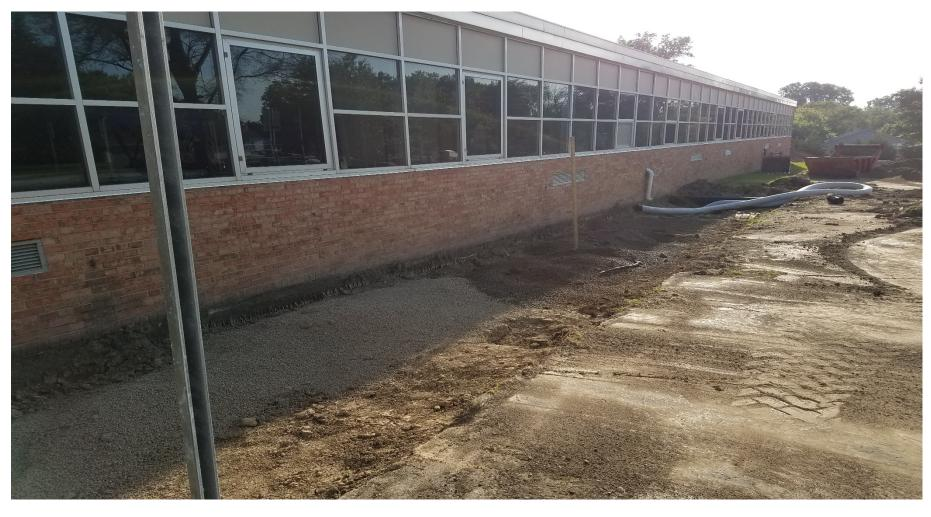
Installation of perforated drainage piping to collect water runoff from the existing school.
