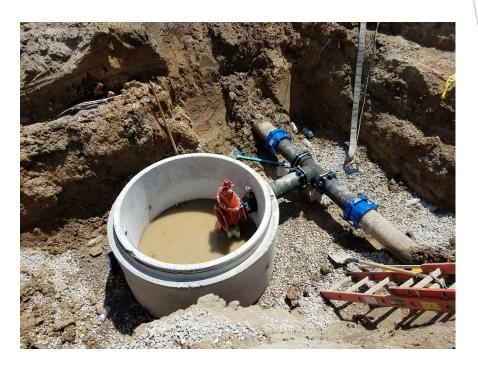
Installation of gate well structure for hydrant water piping.
