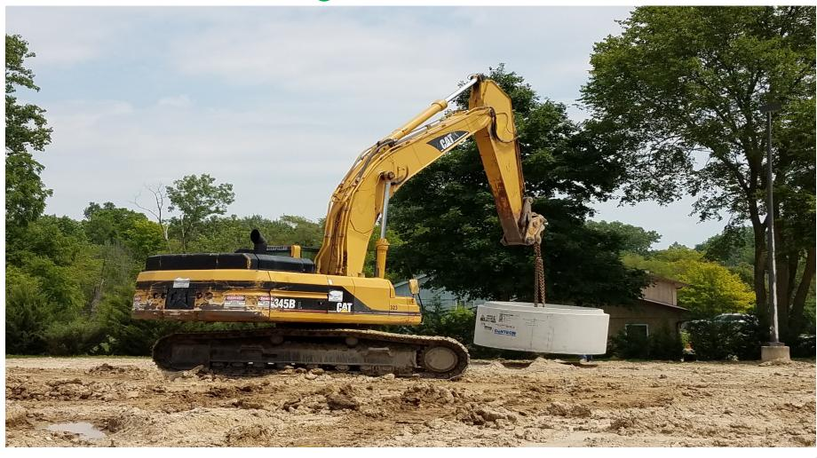
Unloading Oil Separator for new detention system.
