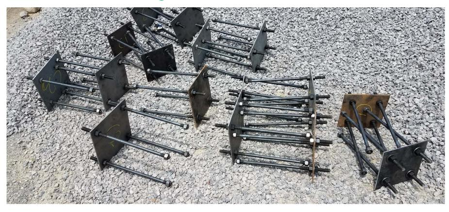
Structural steel base plates for embedment into concrete foundations.
