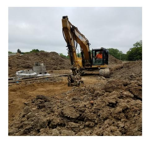
Sand backfill and compaction of storm piping.
