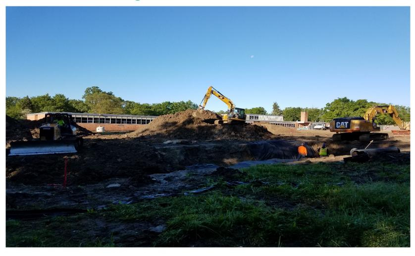
Earthwork equipment working in tandem to install underground piping and structures.
