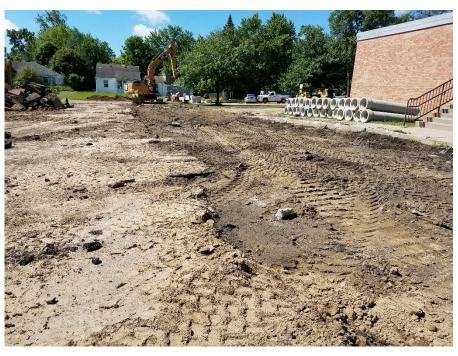
Removal of parking lot for underground piping and structure installation.
