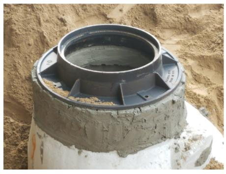
Setting man hole structures to grade: Before and After.
