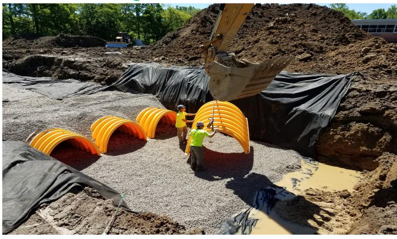
Installing final sections of underground storm detention system.
