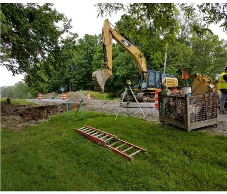
Water tap into existing water main for install of new fire hydrant.
