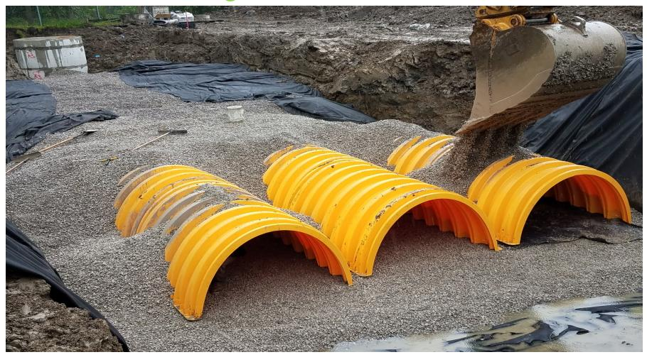
Installation of underground storm water detention system underway.
