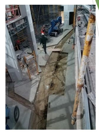
The drywall work in the auditorium is well underway along with the underground electrical work for the new audio/visual control from the new control booth and directors booth locations.
