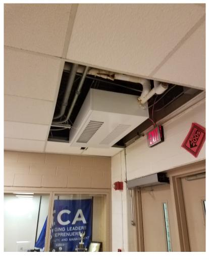
The unit heaters throughout the building are being replaced and the lighting in the auxiliary gym and auto shop was replace over winter break.
