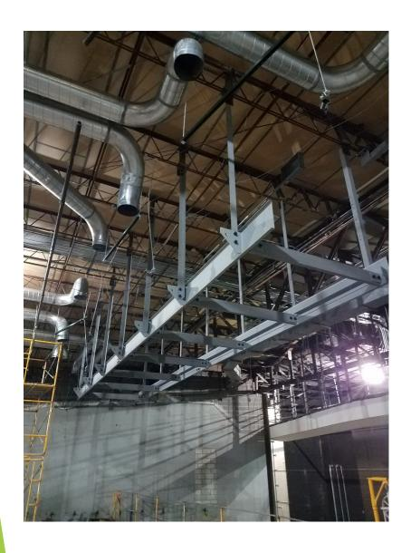
The old catwalk has been removed and the new one is being installed. It was difficult to walk along the old catwalk due to the confined height and width; the new one provides 6' head clearance and 6' width, allowing much improved access.
