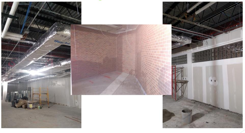
The rough Mechanical and electrical work in the Media Center is complete as well as the glass block along the office wall and the thin brick in the café area.
