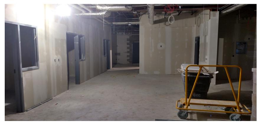
The new Main Office area is well under way as the drywall is ready for sanding and paint.
