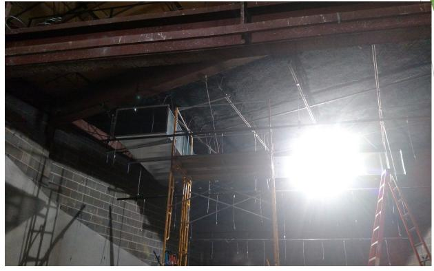
In the Auditorium demolition is nearing completion as the existing catwalk is being removed to make way for the new one. New Mechanical and electrical systems are underway as well.
