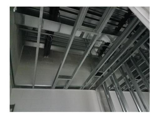
Above ceiling piping and ceiling framing underway.
