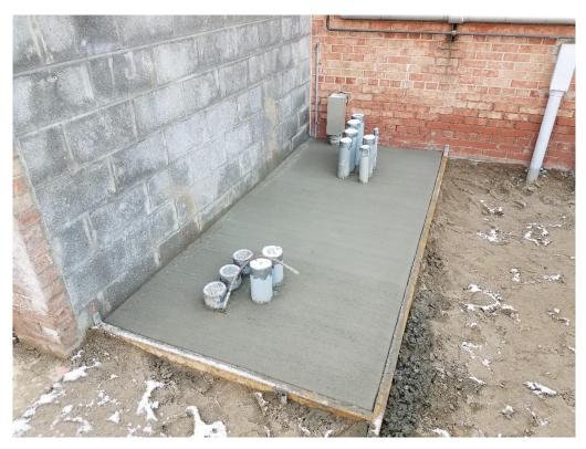
Concrete pads for new electrical service and generator.
