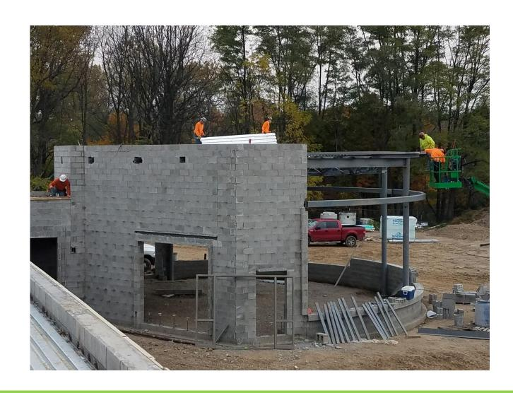
Ironworkers installing joist and metal decking.
