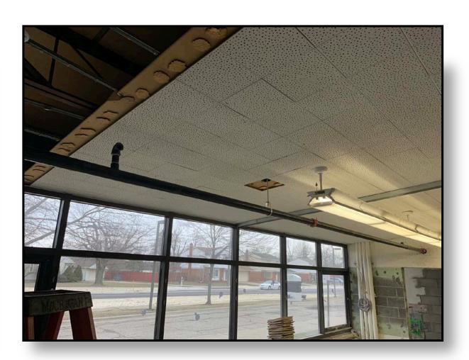
New fire suppression piping is currently being installed.
