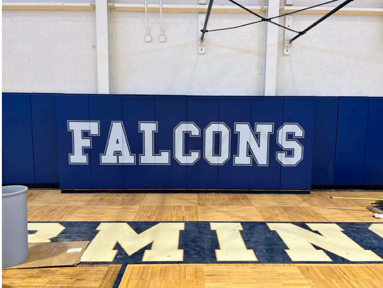
New gymnasium wall pads have been installed
