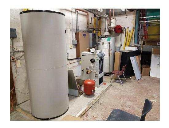
New water heater install in progress (existing water heater to be replaced in background).
