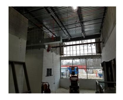
Plumbing, mechanical, electrical pipe and systems installed above ceiling.
